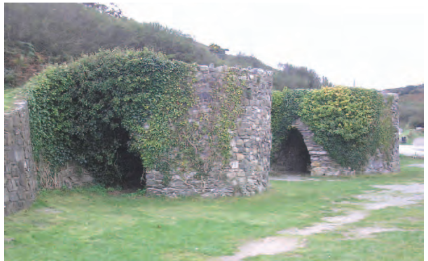
Figure 20.6 Lime kilns. Used to ‘burn’ (heat) chalk or limestone (calcium carbonate) to produce quicklime (calcium oxide)
