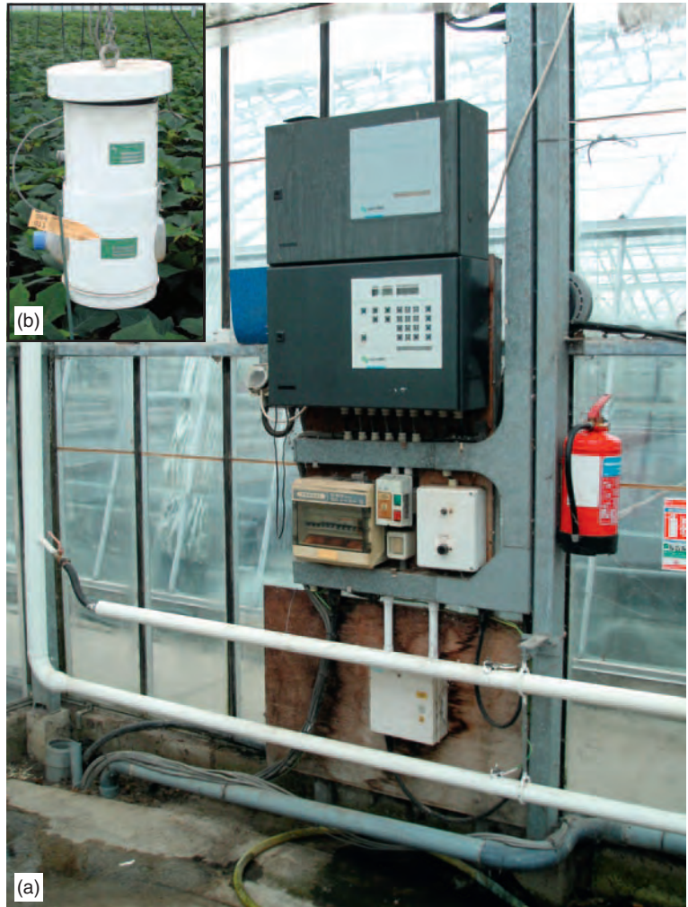
Figure 8.7 The glasshouse environment may be controlled by means of (a) a computer situated in the glasshouse, while (b) conditions are monitored throughout the glasshouse
