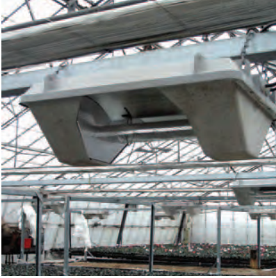
Figure 8.6 High-pressure sodium lamp is used for supplementary lighting
